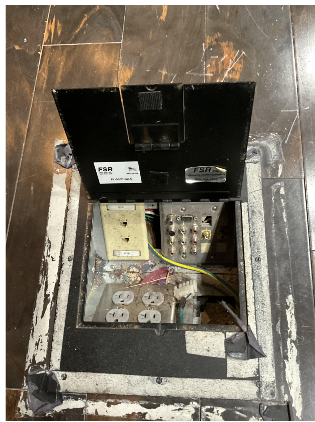
3 STAGE BOX (TYP.) SCALE: NONE
