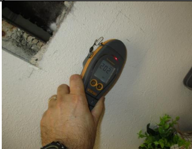
Photo 9: South restroom – tested location of plaster wall at reported plumbing leak location measured dry (202 REL)
