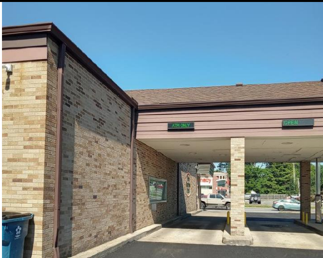
Photo 1: View of drive-thru teller exterior location
