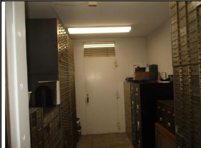
Photo 15: Center vault – overview
