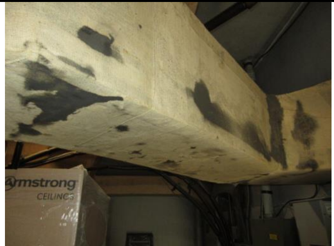
Photo 20: HVAC closet – example of main trunk line exterior insulation (negative for asbestos)
