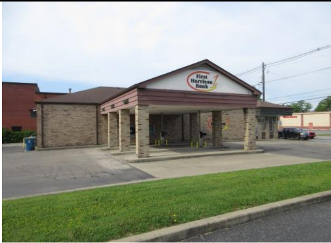
Photo 1: Subject property overview – 130 S Buckman Street, Shepherdsville, KY – front (north) elevation
