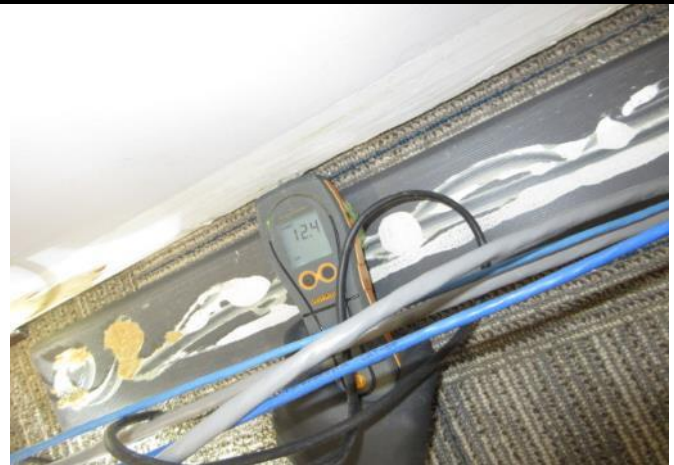
Photo 8: Tested location of exposed drive-thru teller office north wall measured dry (< 16% - typical)
