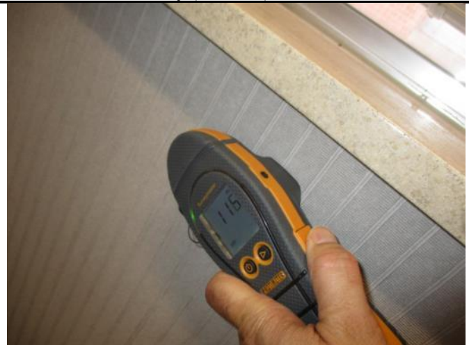
Photo 16: Lobby – tested location of wall below typical window measured dry (115 REL)
