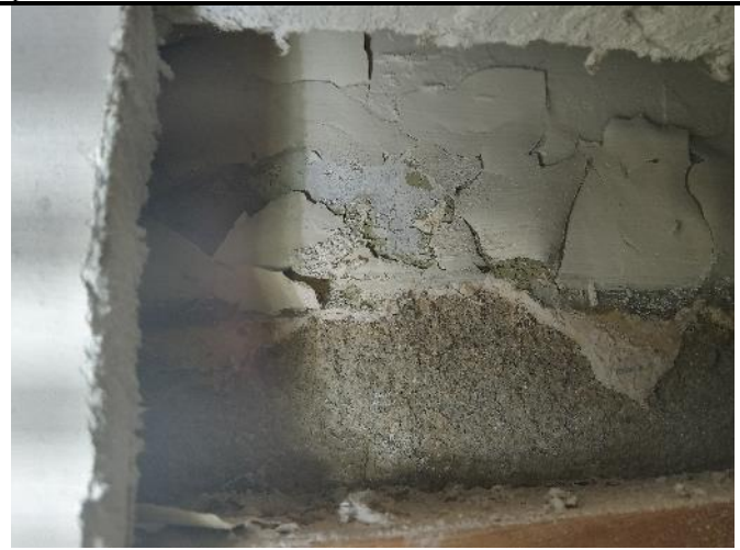
Photo 12: Exposed location of north wall cavity appears generally clean (as viewed through view hole)
