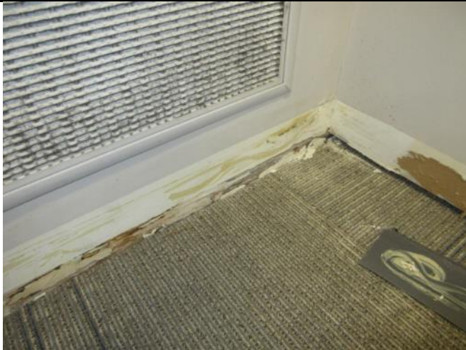
Photo 9: View of drive-thru teller office west wall below HVAC return air inlet
